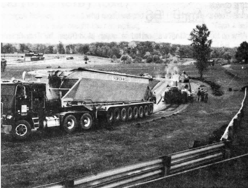
Work crews apply a new asphalt surface to turn four, Hilltop Turn, in front of the spectator bleachers at Waterford Hills Race Track. The 1.5 mile road course is host of the annual Meadow Brook Historic Races, scheduled for Aug. 5-7 this year. [ MOTORSPORTS PROMOTIONS - PHOTO ]
